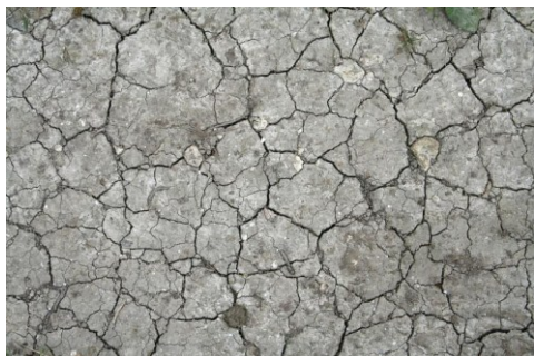
Slika 7. Ispucala glina. Figure 7. Cracked clay.
