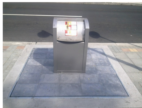
Figure 1. Underground containers – capacity 3 m 3 .
